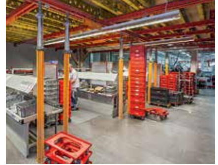
Inexpensive supporting structure consisting of MULTIPROP Props in combination with VARIOKIT system components.
