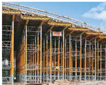
MULTIPROP Shoring Towers as sub-structures for project-specific slab tables.
