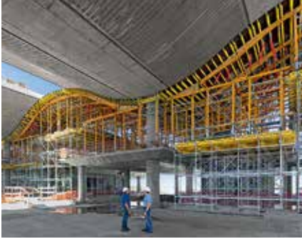
VARIOKIT and MULTIPROP system components formed the cost-effective basis for the form-shaping slab tables.
