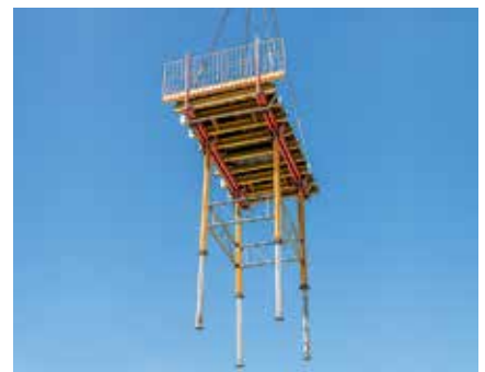
With VARIODECK Tables, the MULTIPROP Props are fixed in their designated perpendicular positions by means of MRK Frames.
