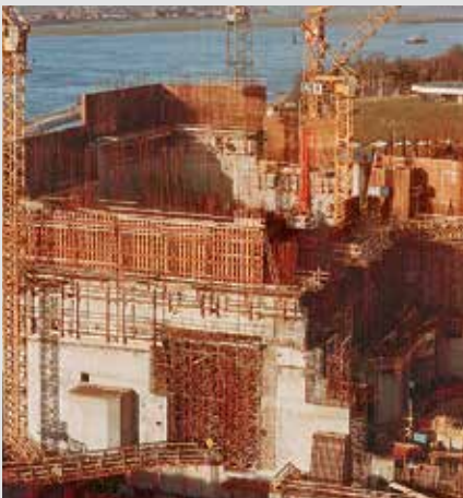
1974 Kümmel Nuclear Power Plant, Germany (KGF, VARIO GT 24)
