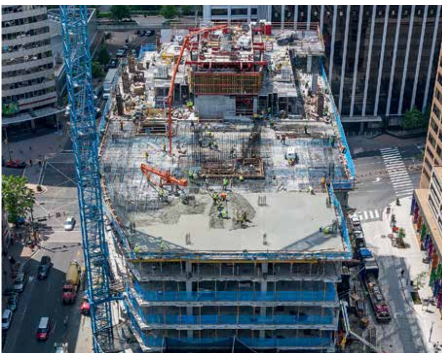
With the ACS Core 400, walls and slabs can also be concreted in one pour. For this, very large placing booms are used.
