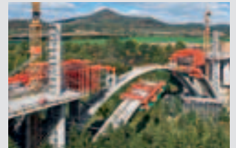
Bridge Formwork
