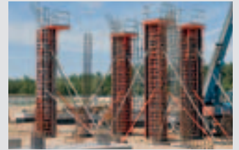
Column Formwork
