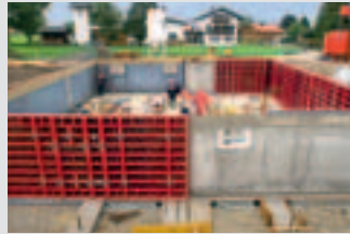
Wall Formwork
