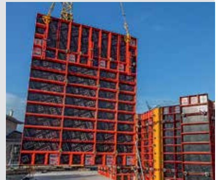
Extensions up to heights of 3.85 m are possible with horizontal LIWA panels. The compensation waler provides the required transfer of forces as well as bracing.
