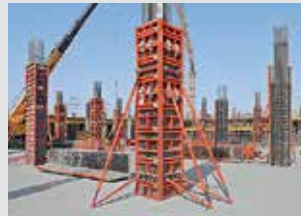
Column Formwork
